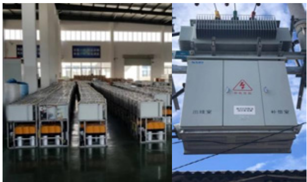
State Grid JiangSu Electric Power Co., Ltd SVG
