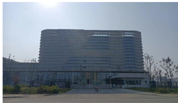
Chengdu Intelligent Computing Center AHF&SVG
